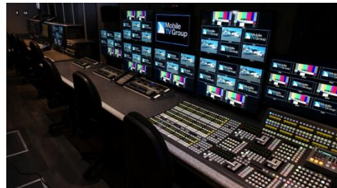
36VMU (B Unit) Production – Kayenne Switcher
